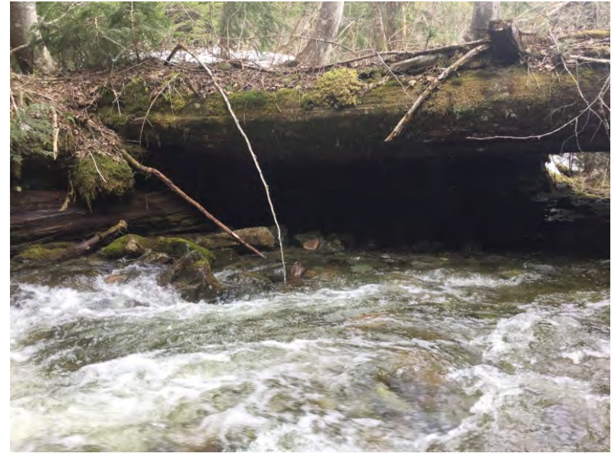
Left Bank Abutment when facing downstream
