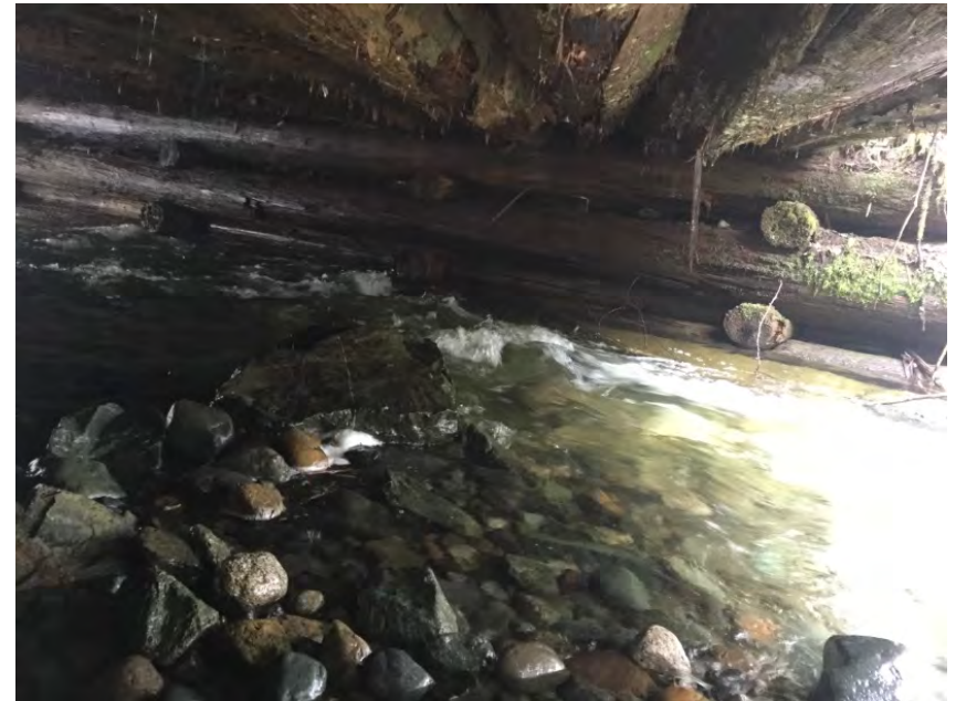
Right Bank Abutment when facing downstream
